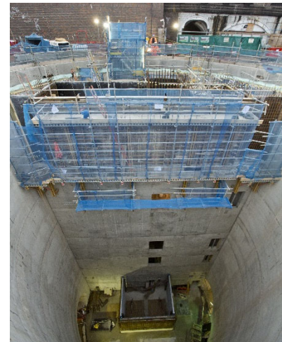
Eleanor Street Shaft
