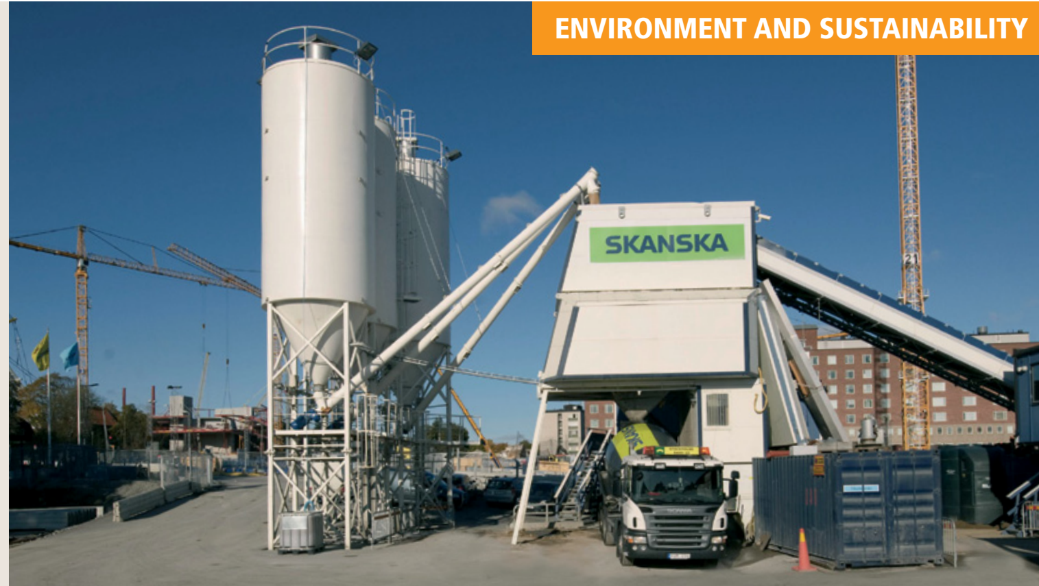
The concrete plant established on the construction site provides the project with concrete and reduces the number of trips by a total of 20,000.
