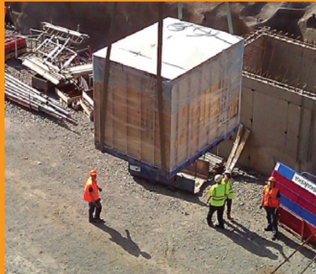
The modules, lifted into place using cranes, are sealed until they are put into use.
