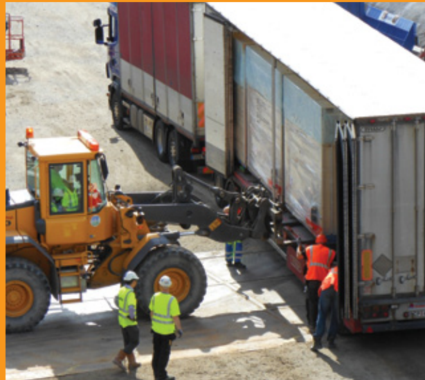
Prefabricated sanitary rooms are delivered as boxes.
