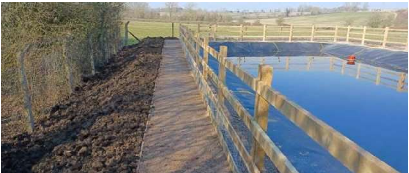
Scrape and liner
