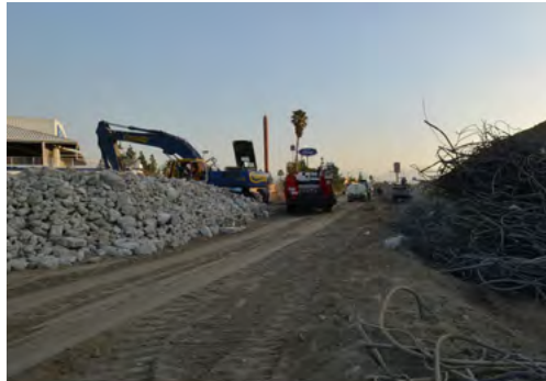
Interstate 215 Widening Project
