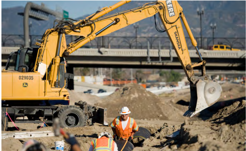
Interstate 215 Widening Project
