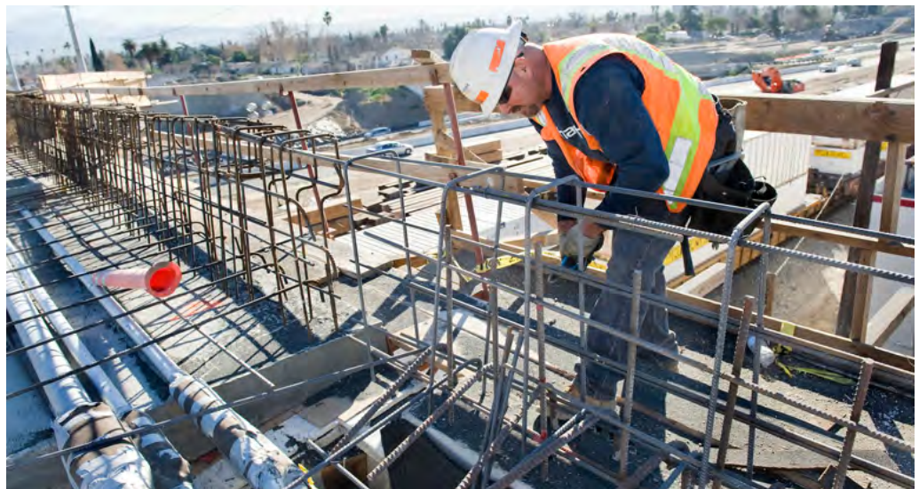
Interstate 215 Widening Project
