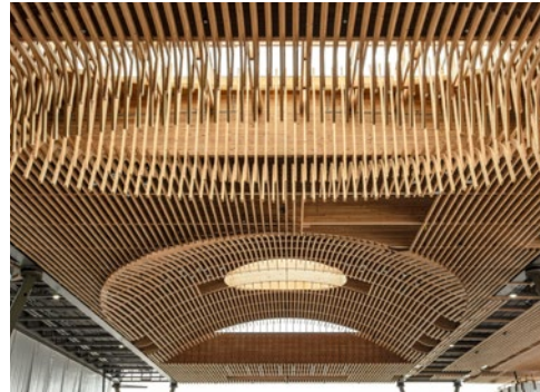
Portland International Airport, Oregon, USA A mass-timber marvel. Page 21
