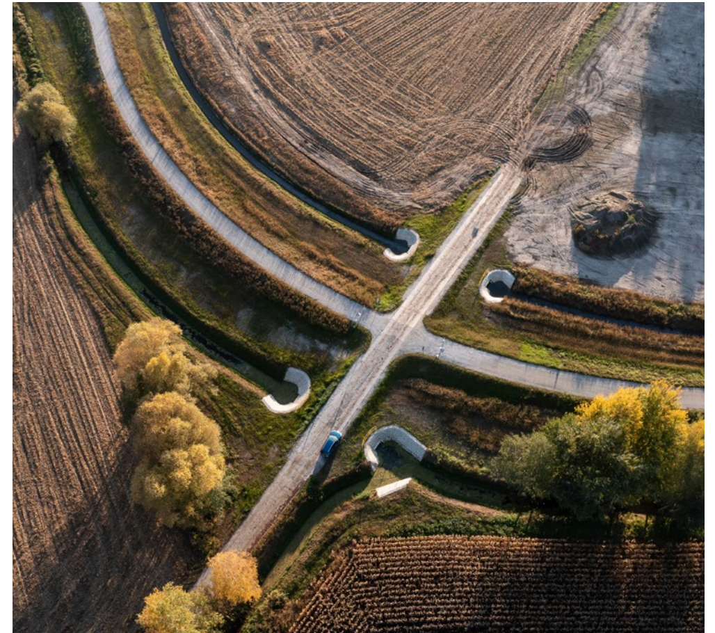
In the city of Wrocław, Poland, which was hit by a devastating flood in 1997, we have modernized the flood protection embankments of the River Widawa to protect the population from future floods. This project was completed in 2023.
