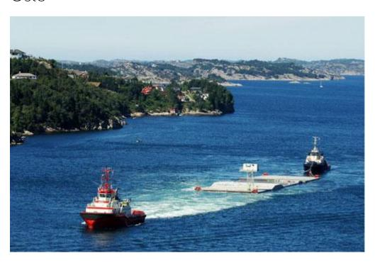
**Immersed tunnel** Costumer: The Norwegian Public Road Authorities Type of contract: Construction and Installation Construction period: Aug 2005 to Dec 2009 Technical data: Length immersed tunnel: 675 meter Six tunnel elements: 112,5 meter in five segments, each 22,5 meter. Width immersed tunnel: Varying, 28-43 meter. Height immersed tunnel: Varying, 9,30-9,80 meter.
