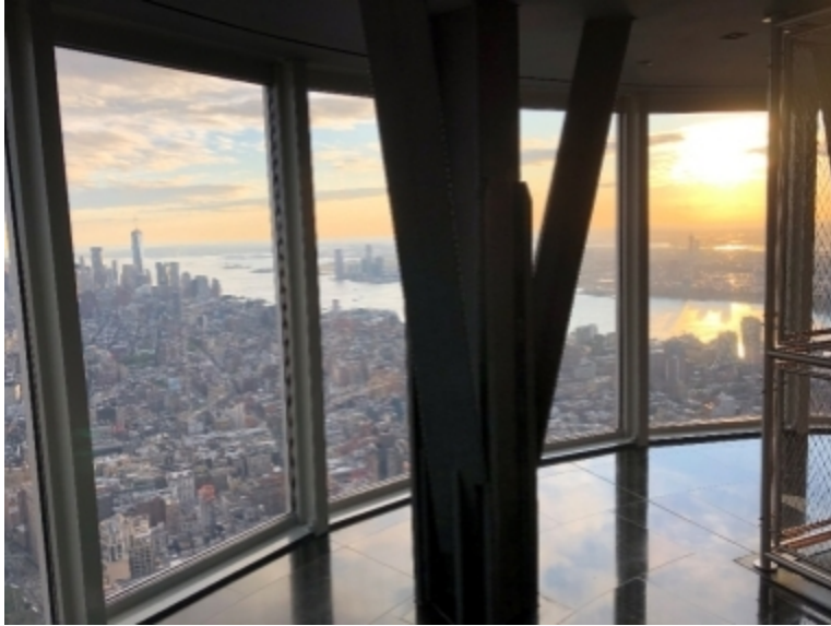
Caption: Skanska replaced the 102 nd Floor Observatory windows with 360-degree floor-to-ceiling windows offering unobstructed, panoramic views of the city.
