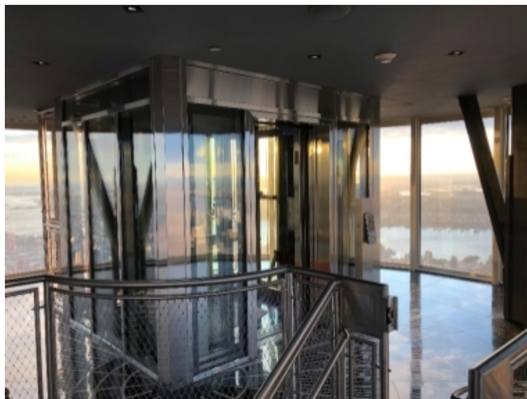
Caption: Skanska installed a brand-new Otis elevator system with an all-glass cab and elevator shaft equipped with technology to provide riders with an immersive experience. The new system affords passengers a panoramic skyline view as they rise to the Observatory level.
