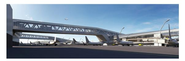
The first of its kind in the world, LaGuardia Central will feature dual pedestrian bridges spanning active aircraft taxi lanes, allowing for improved aircraft circulation and gate flexibility.
