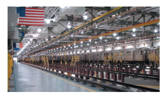
passenger cars along the number 7 subway route. The facility is better designed with wider service aisles between tracks and sufficient ceiling height for an overhead crane, which facilitates moving material and equipment. The facility is also equipped to support car modification programmes and to more effectively service modern models of passenger cars.
