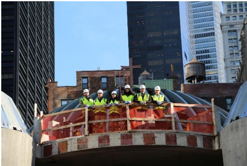
Photo 1 Caption: Skanska USA team members celebrate the topping out of the St. Nicholas Greek Orthodox Church and National Shrine, representing the completion of the structural steel erection at the site.
